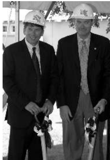
Assemblyman Sean Kean and Freeholder Robert Clifton get ready to break ground.
