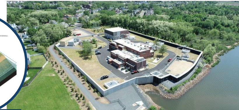
Sayreville Pump Station, Sayreville NJ
