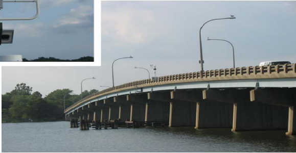
Sensors at Gooseneck Bridge Location
